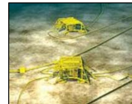
Raw Seawater Injection
