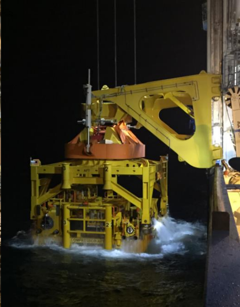
Compressor Module #2 deployed 8th September 2015 in Hs 2.5m
