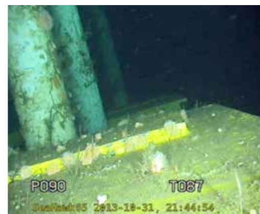
Example of a SeaHawk(tm) video picture from an installation.
