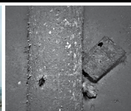
Debris near the pipe.
