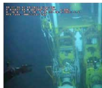
View of xmas tree with both lines connected.
