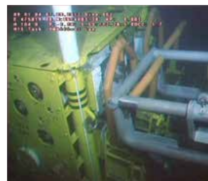
Landing of first end of flexible into porch.
