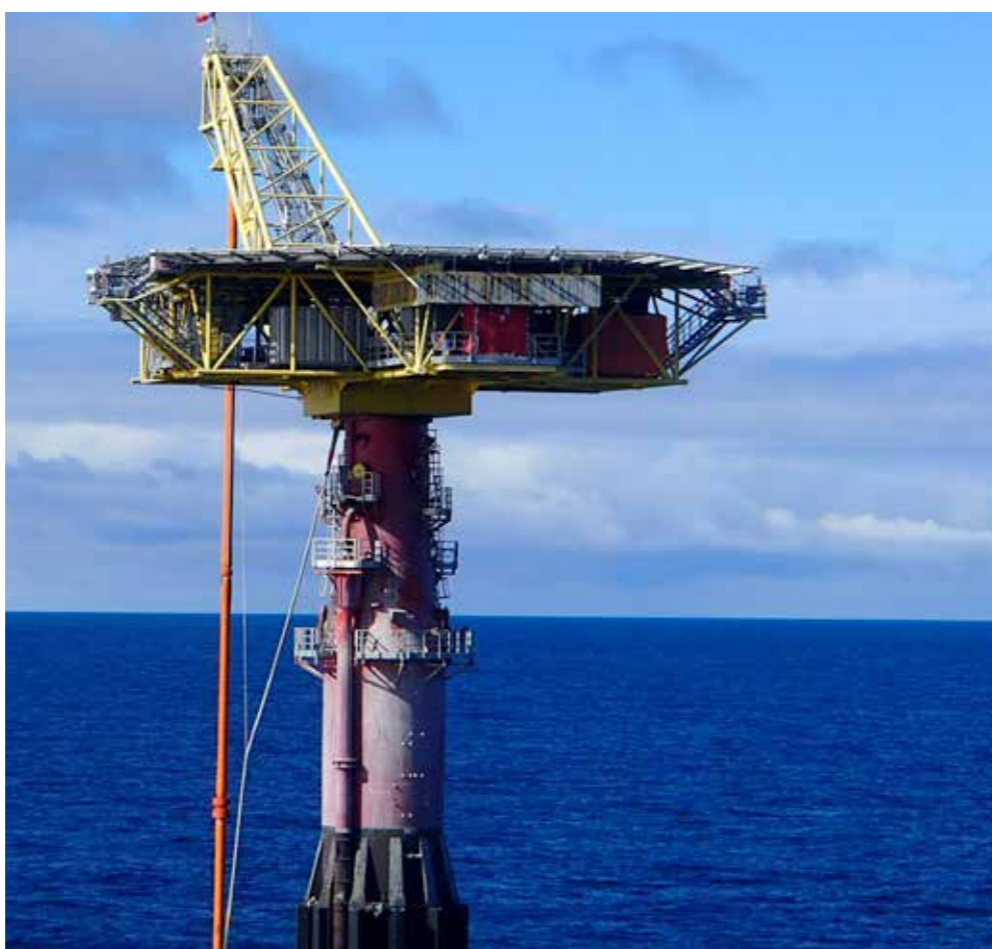
Draugen Floating Loading Platform.
