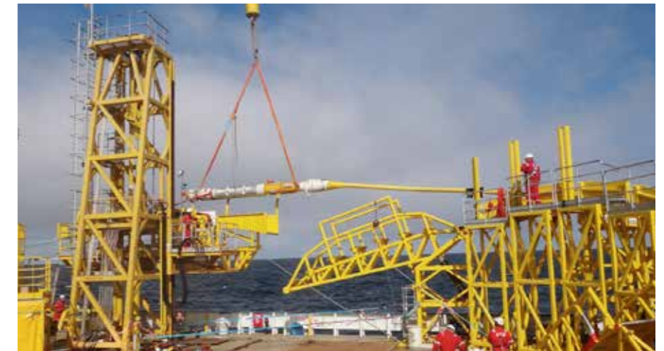
Static end termination handling onto support track
