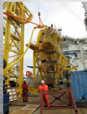
Transition joint deployment
