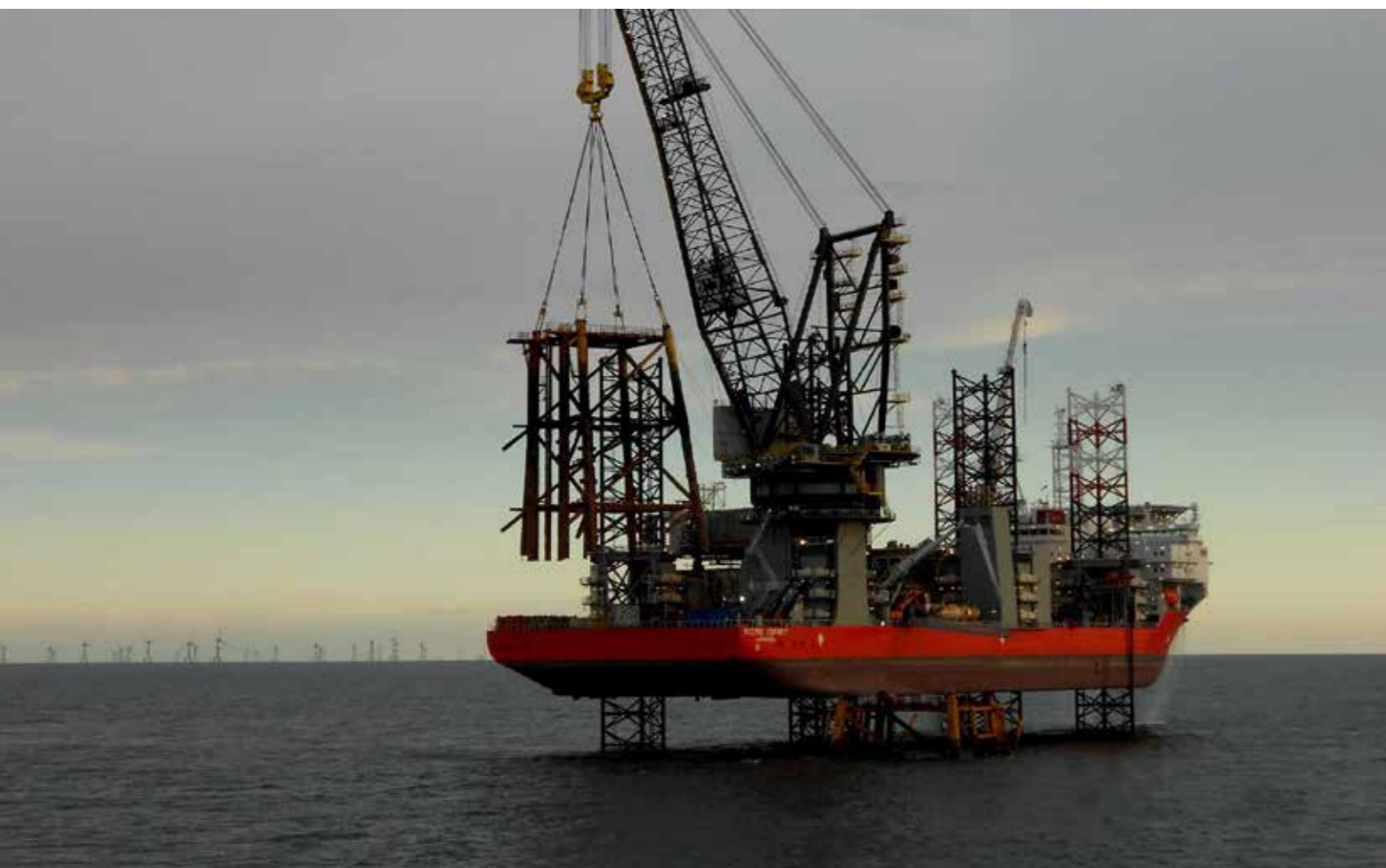
Lifting of bottom section.
