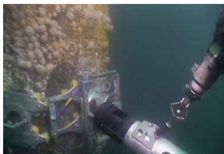
Drilling of 100 mm holes.
