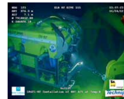
Installation of SPC Aft at Tamp B
