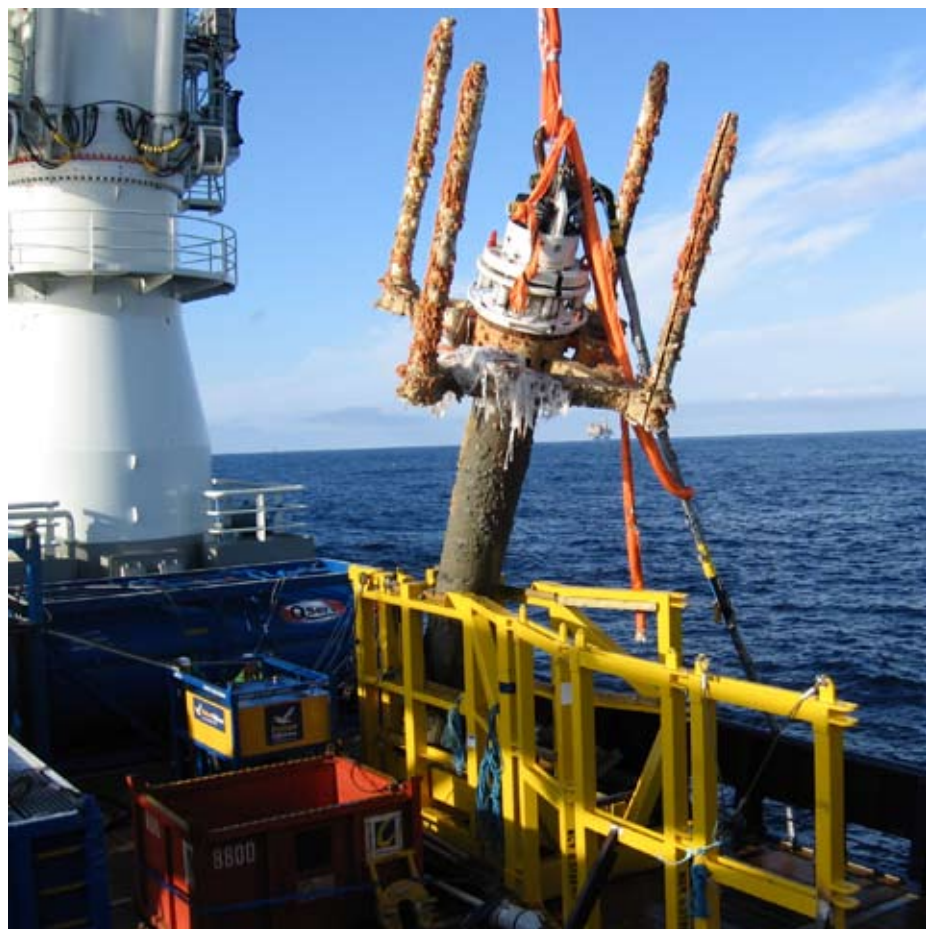
"Subsea wellhead and guide base being safely laid out on deck by the Subsea Wellhead Picker"
