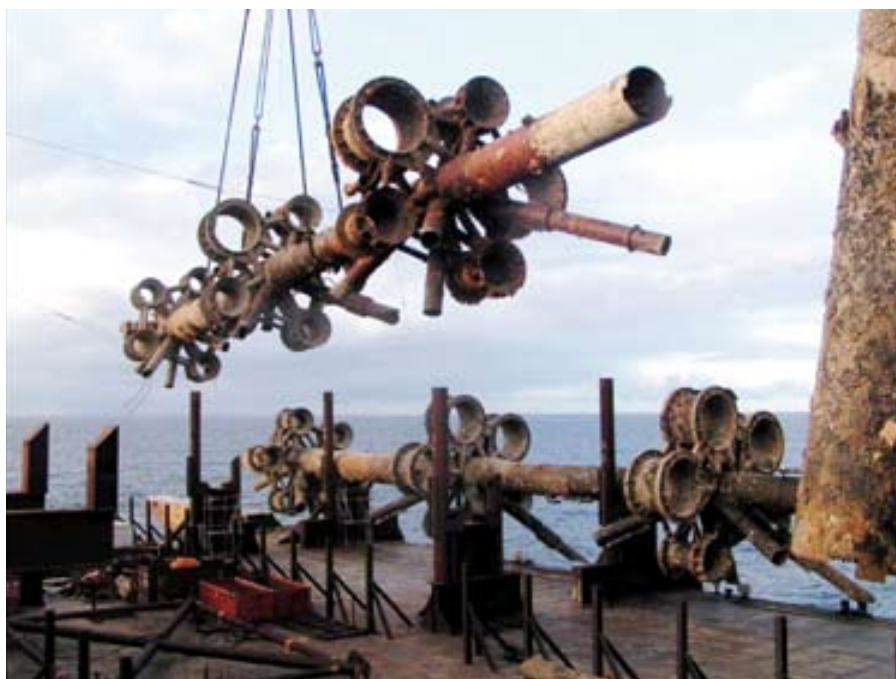
The picture shows "castellated" cuts at the end of the jacket section
