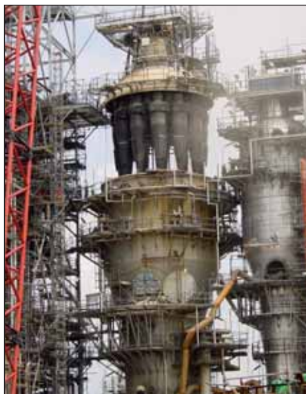
Photo 4 Cracker Internals being lifted
