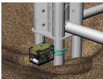
05. WROV installs GR on pile
