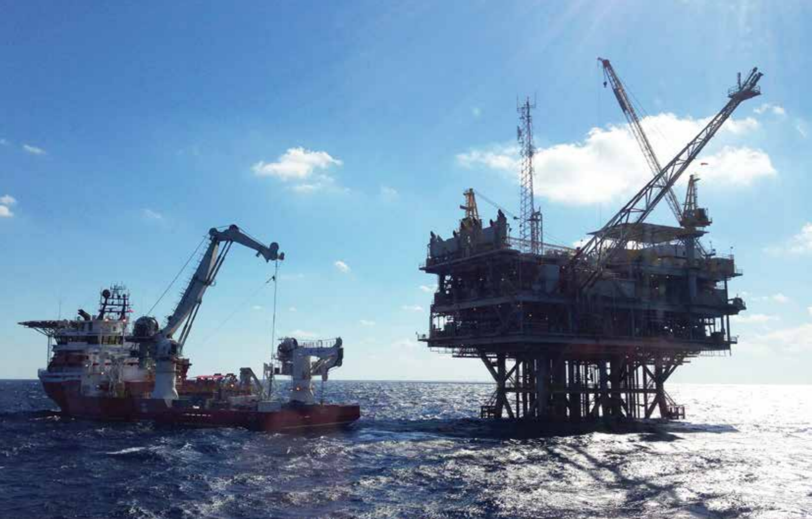
TDW SmartPlug Inline Isolation Tool being positioned for launch.
