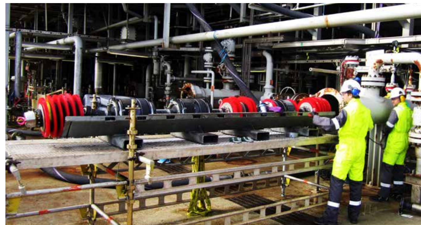
TDW SmartPlug Inline Isolation Tool prior to launch.
