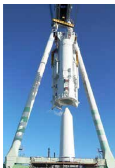
SHS Superstructure being landed on the King Post.
