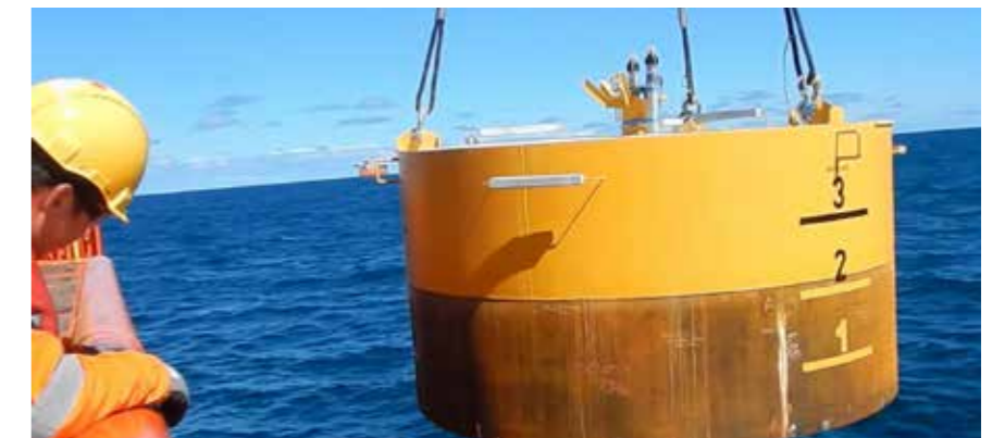
Installation of 170 Te horizontal anchor for Water Injection riser on Heidrun
