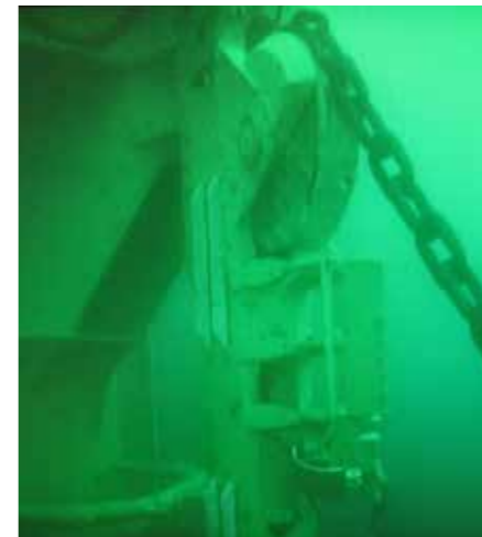
Monitoring pull in of anchor chain.
