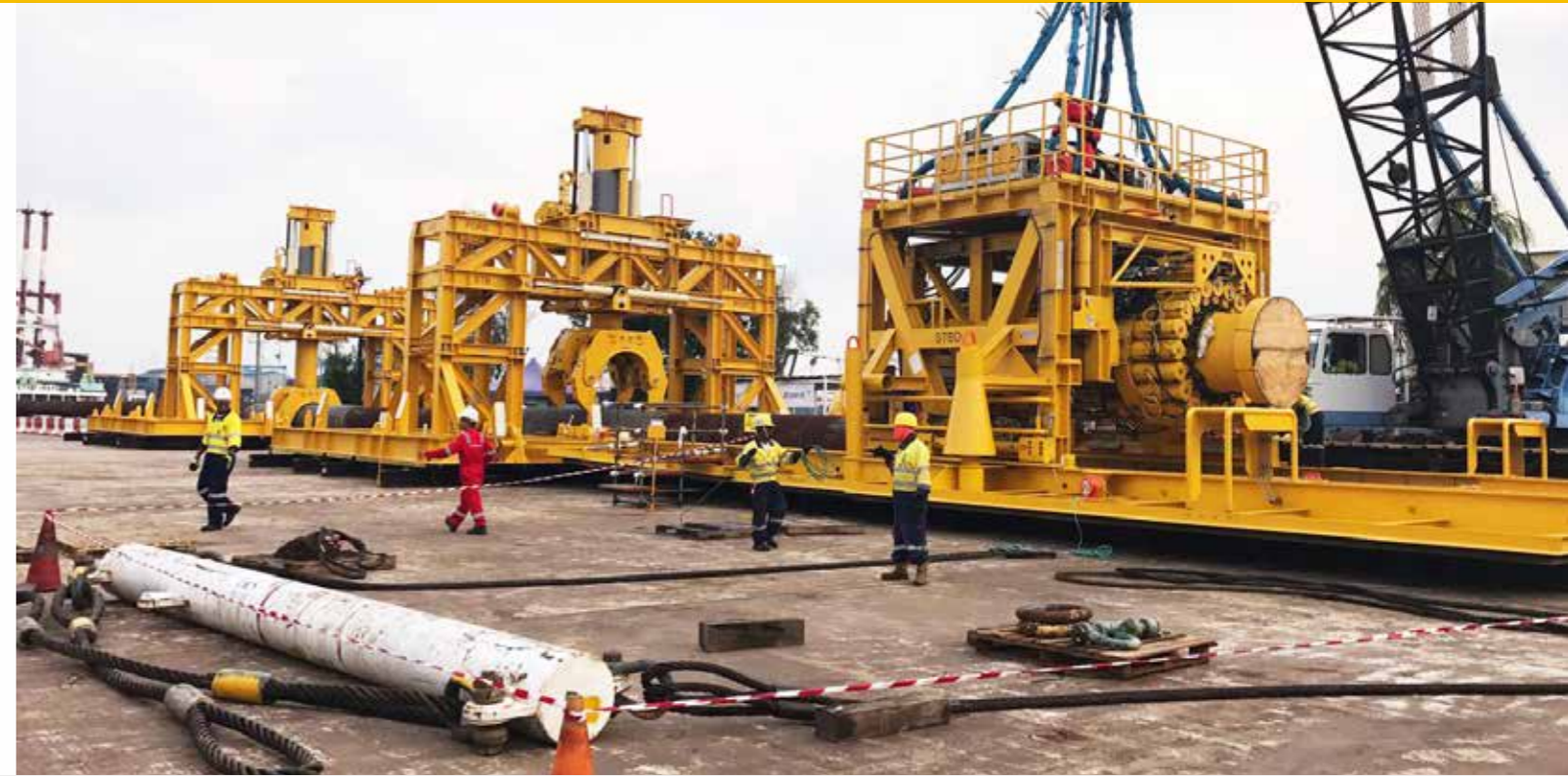
SIT in Singapore - lifting and alignment frames and PFA frame.
