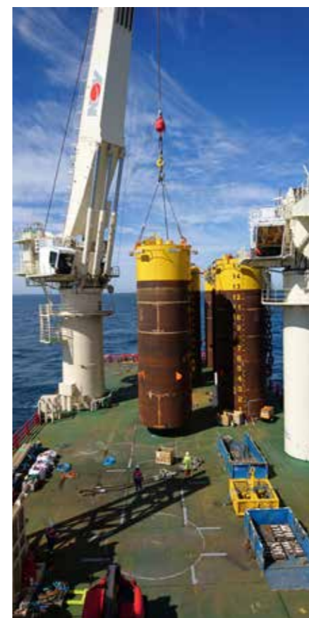
Suction anchor installation.
