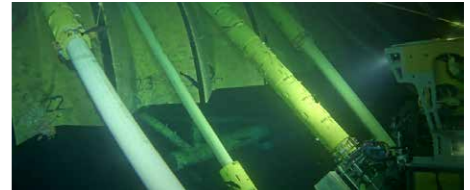
WROV operating push/pull unit to install WPE rack onto RSS
