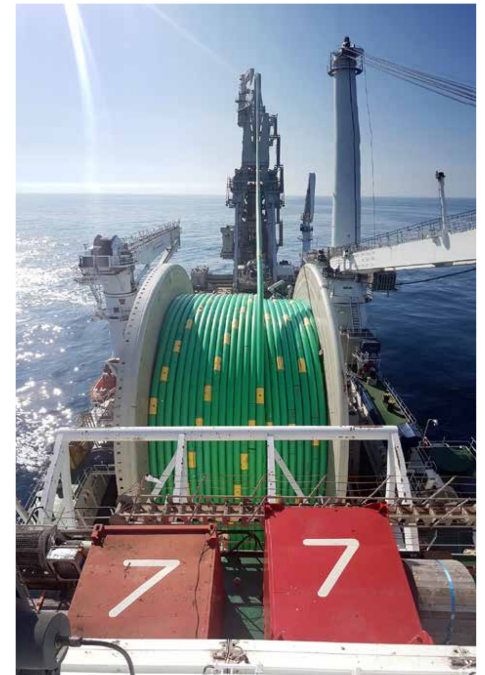
Seven Oceans installing Mechanically Lined BuBi pipe.
