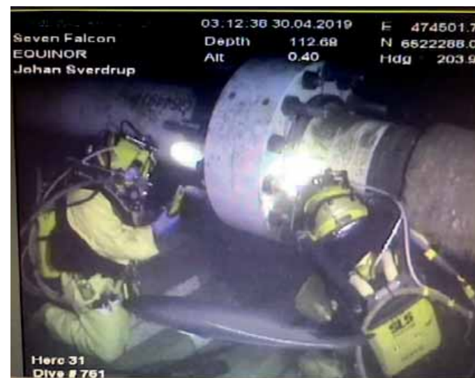
Divers making up an 18" SeAlign flange on Johan Sverdrup
