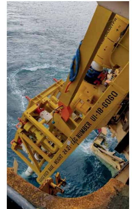
Installation of 10" Bauge PLET/PLR (TechnipFMC) with SeAlign connector
