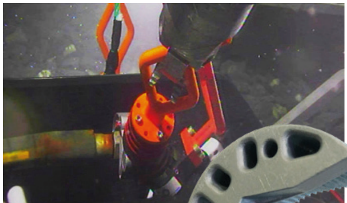
Installation of metal 3D printed clamp subsea.
